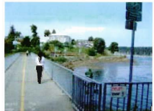
Walkway over the Millstream River
